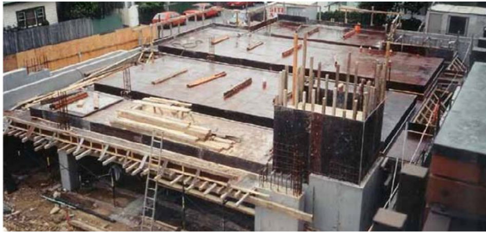
Construction of Sir Eric Pearce House well under way in 1994.
