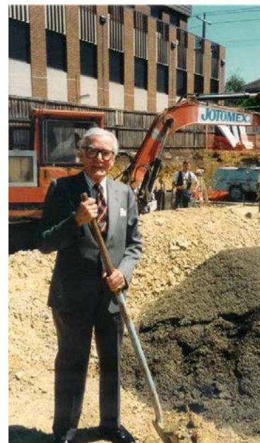
Sir Eric Pearce at the commencement of work on the site for the frail aged hostel named in his honour.
