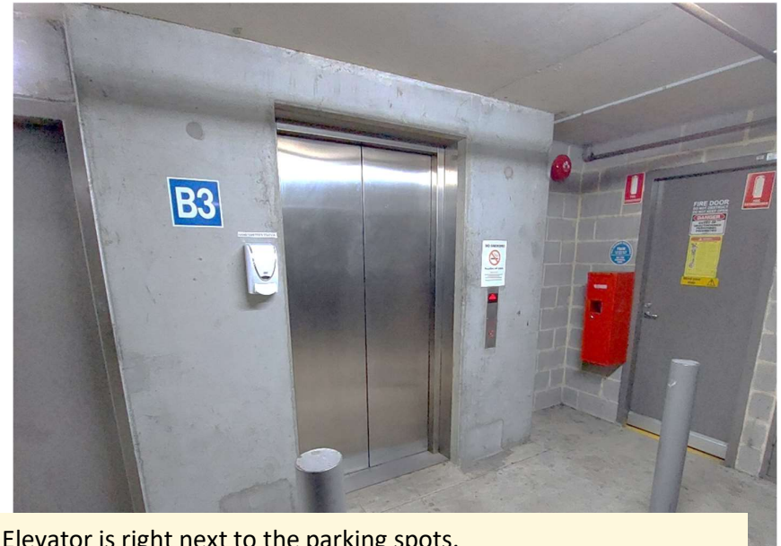
Elevator is right next to the parking spots.
