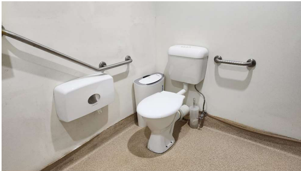
Handrail is on the right hand side when sitting down.
